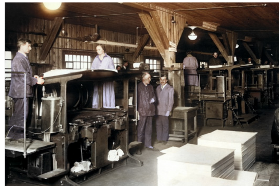
State Printing Works in Warsaw: checking the quality of the paper and watermarks; in the background, banknote printing machines, 1920s / NAC COLLECTIONS
